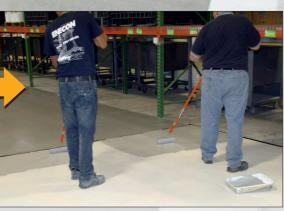
CHEMCLAD® P4C is a two component, water borne, polymeric adhesion enhancer specifically formulated to help seal concrete / cementitious surfaces and insure optimum interface bonding between the surface and the ENECON® High Performance Polymer System selected as the finish coat.
