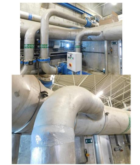
Taking into consideration the corrosive environment, all surfaces were coated with ENECON's CHEMCLAD SC for maximum protection.
