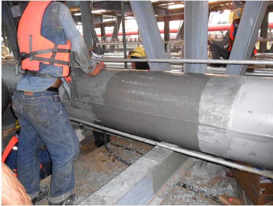
Apply DuraWrap primer for on prepared area.
