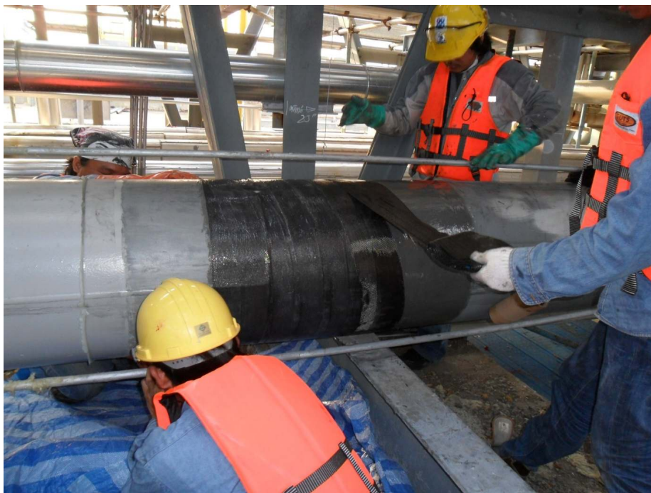
Apply Carbon fiber fabric onto the DuraWrap primer layer.
